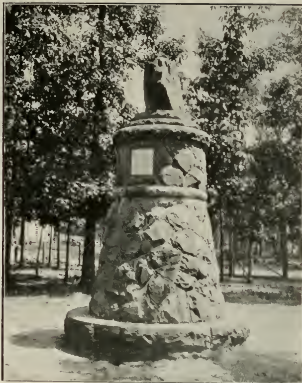
"STANDING STONE" MONUMENT, MONTEREY, TENN.
