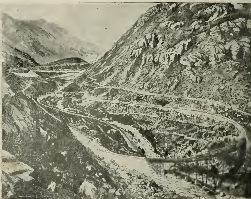
Famous Georgetown Loop, in Clear Creek Canyon. This Railroad Crosses Itself Four Times within One Mile. Robert E. Lee Tunnel is Seven Miles up the Canyon from this Loop.
